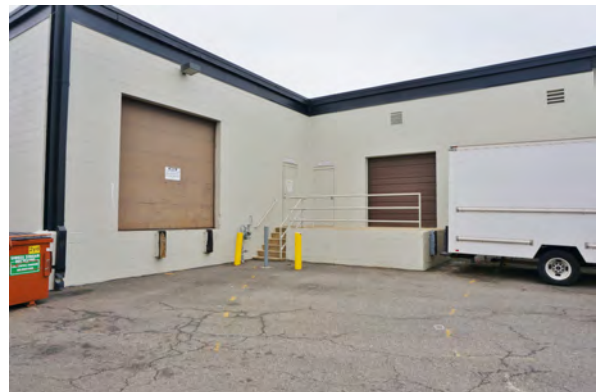
Loading Dock Entrance
