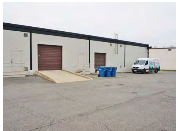
Drive-In Access w/ Ramp
