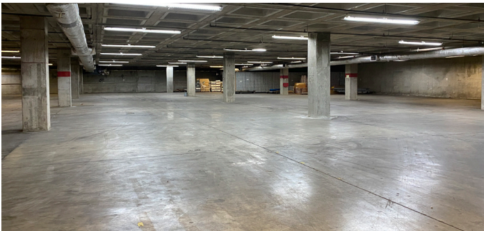
36,500± SF CLIMATE CONTROLLED AREA
