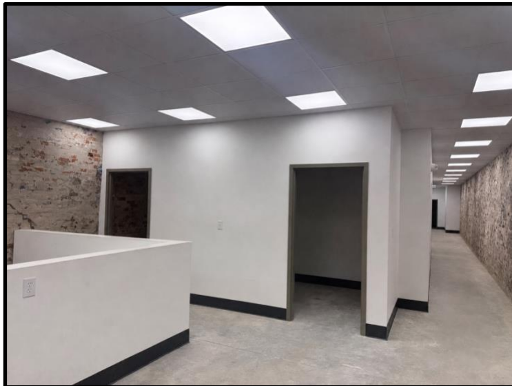
Interior: Restaurant – Partial Bar, Bar Restrooms, Hallway
