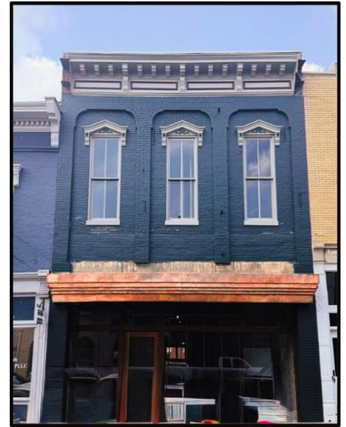
Exterior: Main Street Façade
