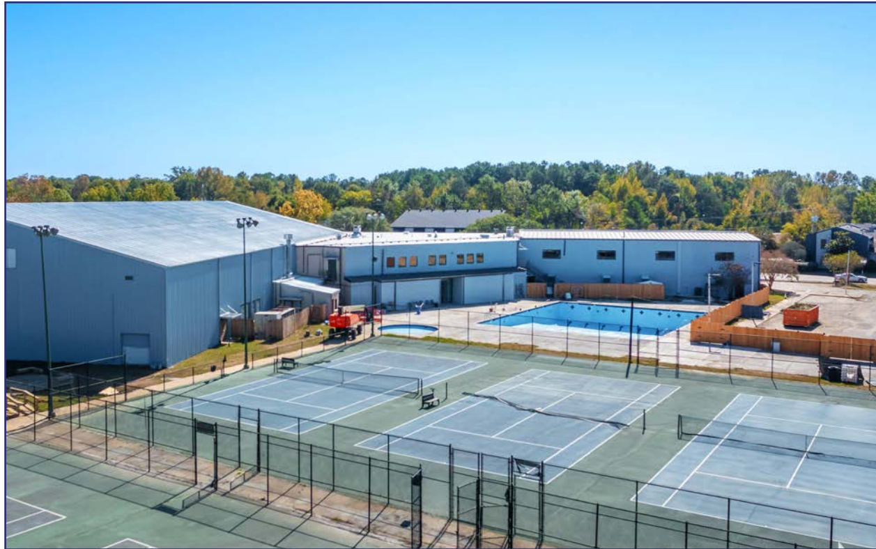
Outdoor Hard-Surface Tennis Courts
