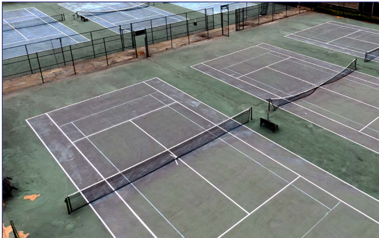
Outdoor Hard-Surface Tennis Courts
