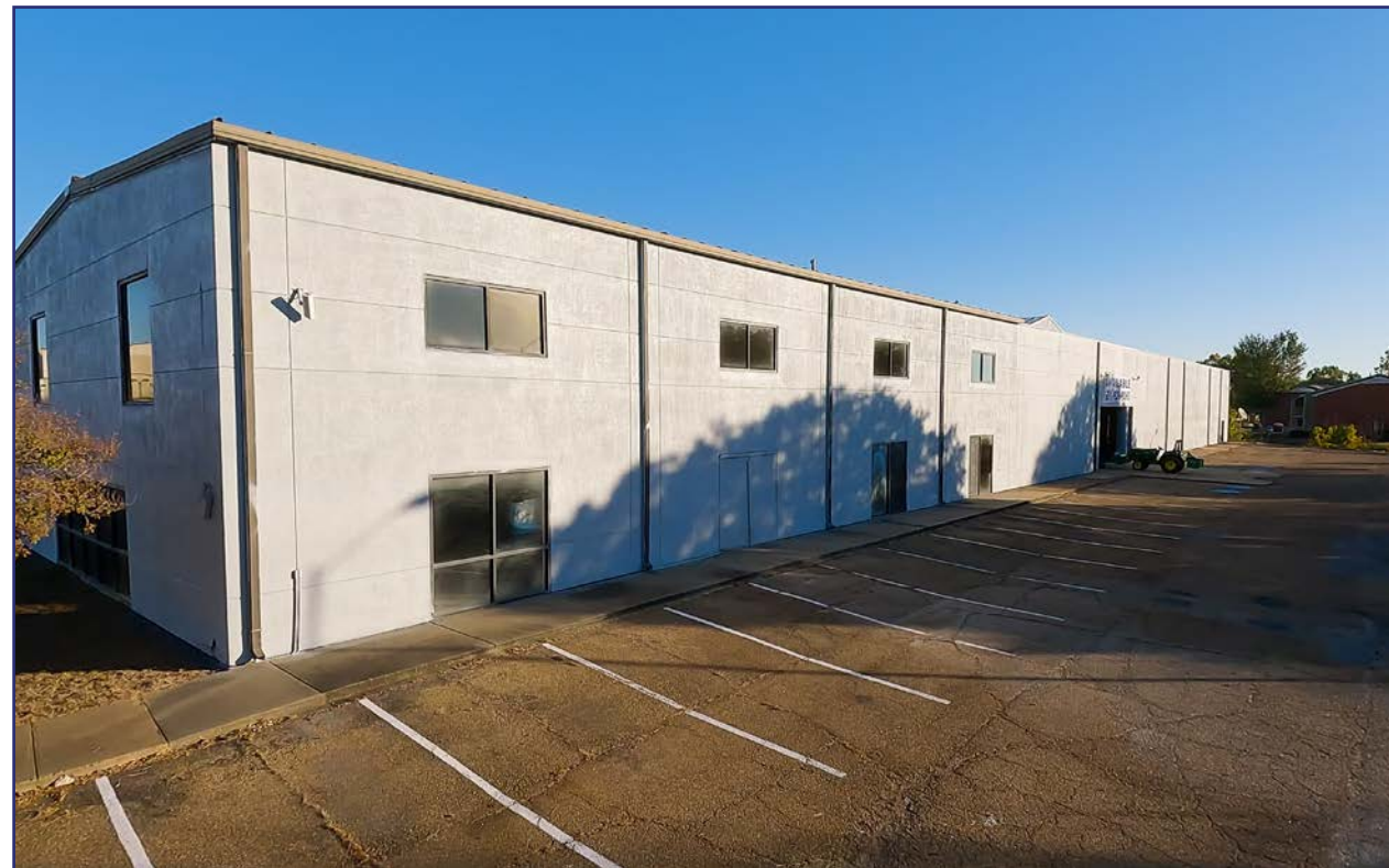
South Parking Lot and exterior facade
