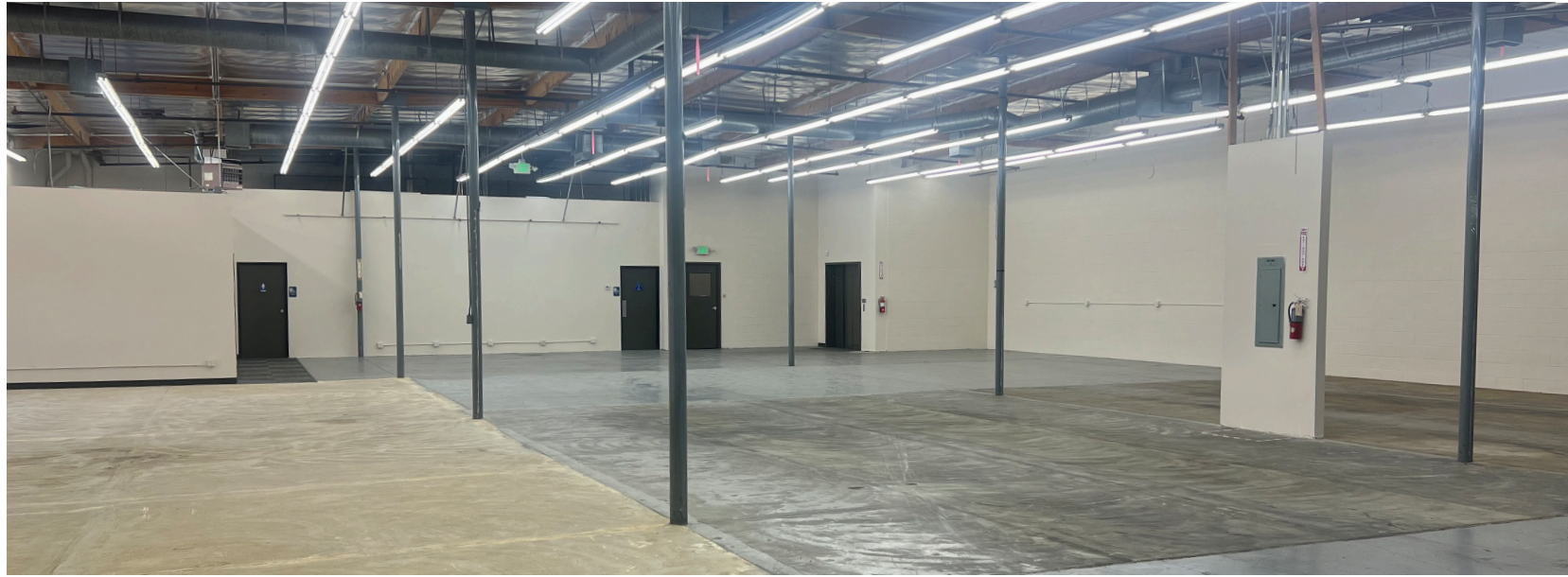
Second Floor Warehouse
