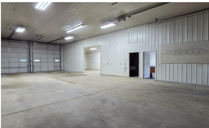
Main Shop / Warehouse
