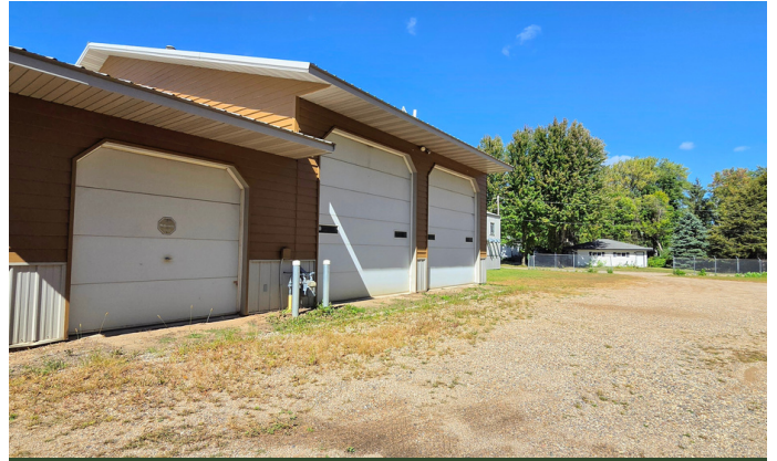
Rear / Overhead Door Access
