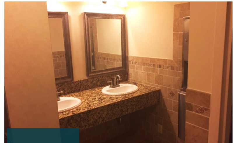
1st Floor Restroom
