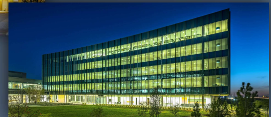
Anadarko Petroleum Building
