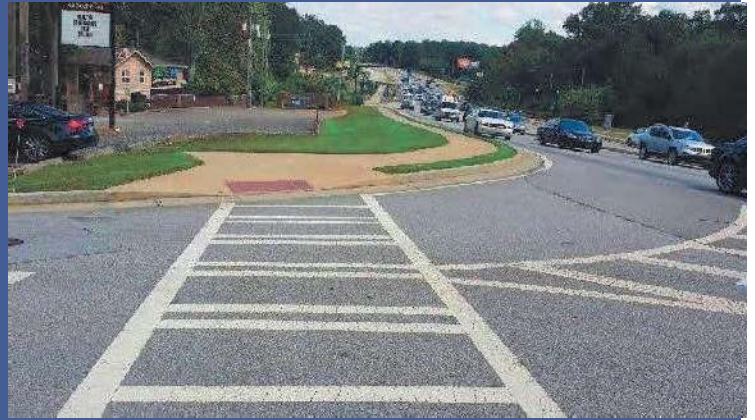
Curb cuts/sidewalks in place
