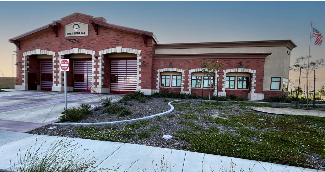
Ontario Fire Station No. 9
