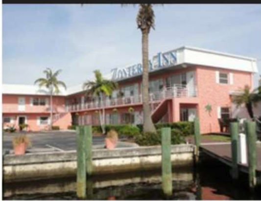
Monterey Inn & Marina 300 SW Monterey Rd. Stuart, FL
