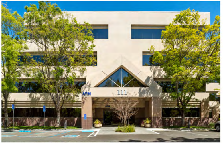
Entrance From Parking Lot
