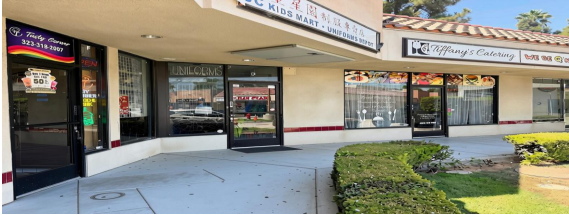
Center Frontage – S. Atlantic Blvd
