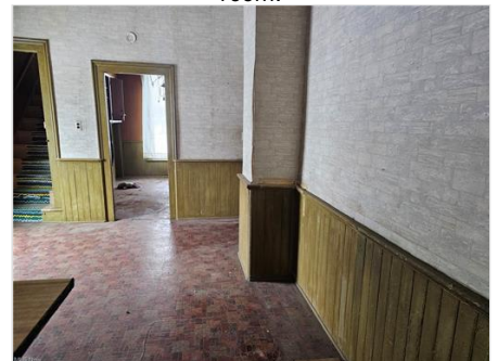
rear west room looking to the front.
