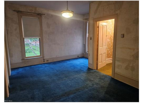
Upstairs Room at the top of the front stairs.
