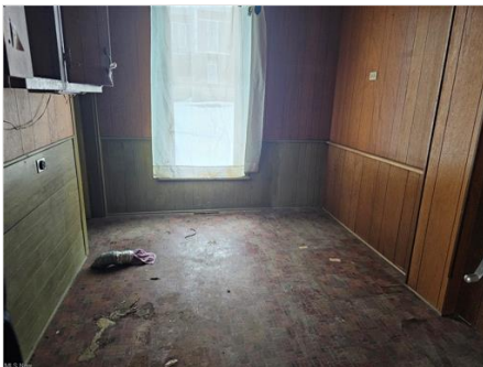
Laundry hookups or a combo pantry storage room off of the kitchen leads to the basement if you need it for deliveries.
