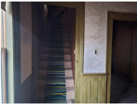
Narrow rear staircase
