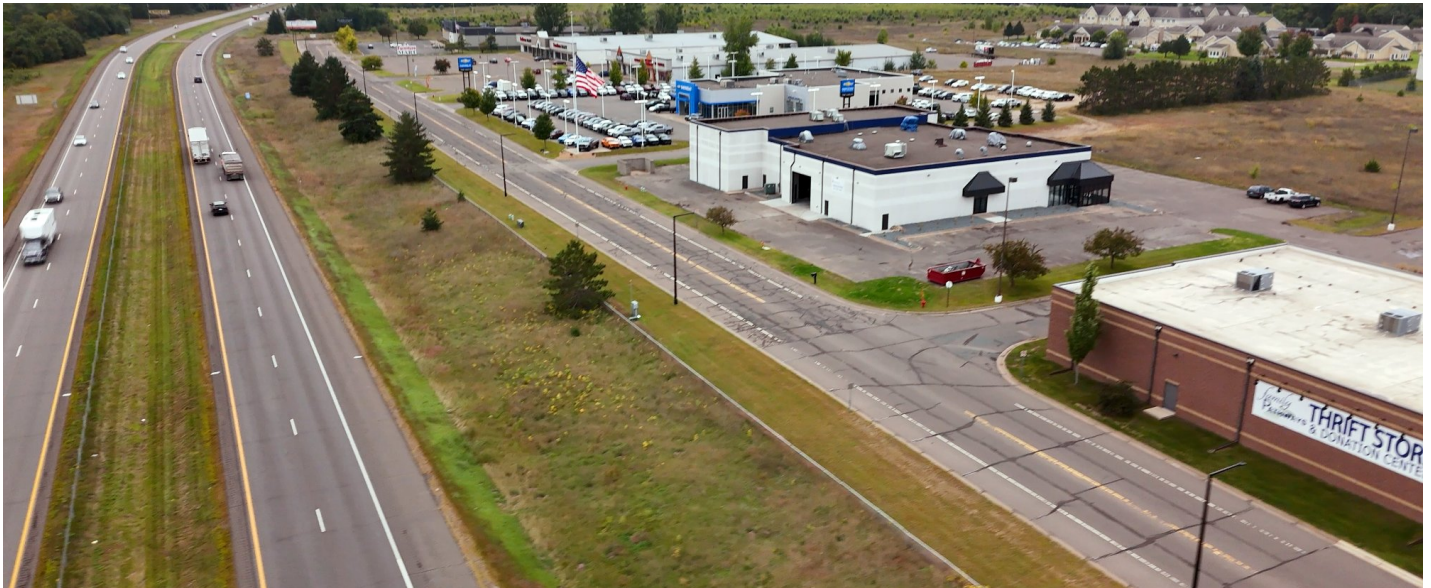
Aerial view showing property's prominent I-35 frontage with excellent visibility and surrounding commercial area
