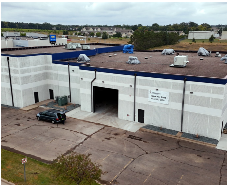
Rear view — overhead door & signage
