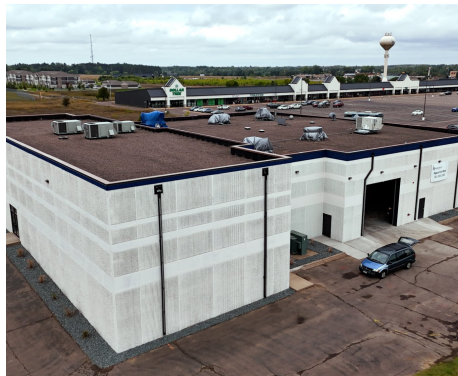
Northeast angle with commercial neighbors
