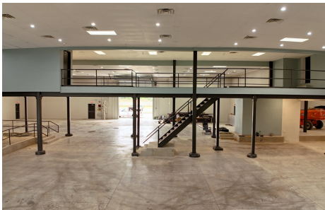
Mezzanine with steel stairs
