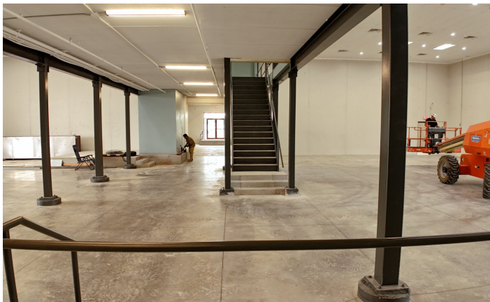
Under-mezzanine workspace with staircase access
