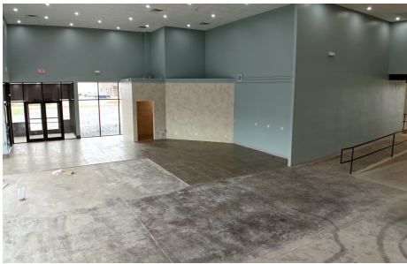
Glass entrance & lobby
