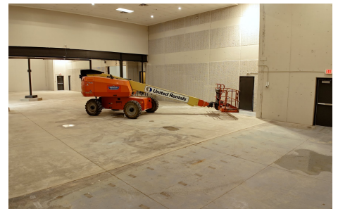
Open floor below mezzanine
