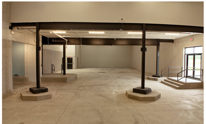
Warehouse area beneath mezzanine with steel beams
