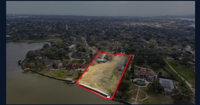
WATERFRONT BULKHEAD — CLOSE VIEW
