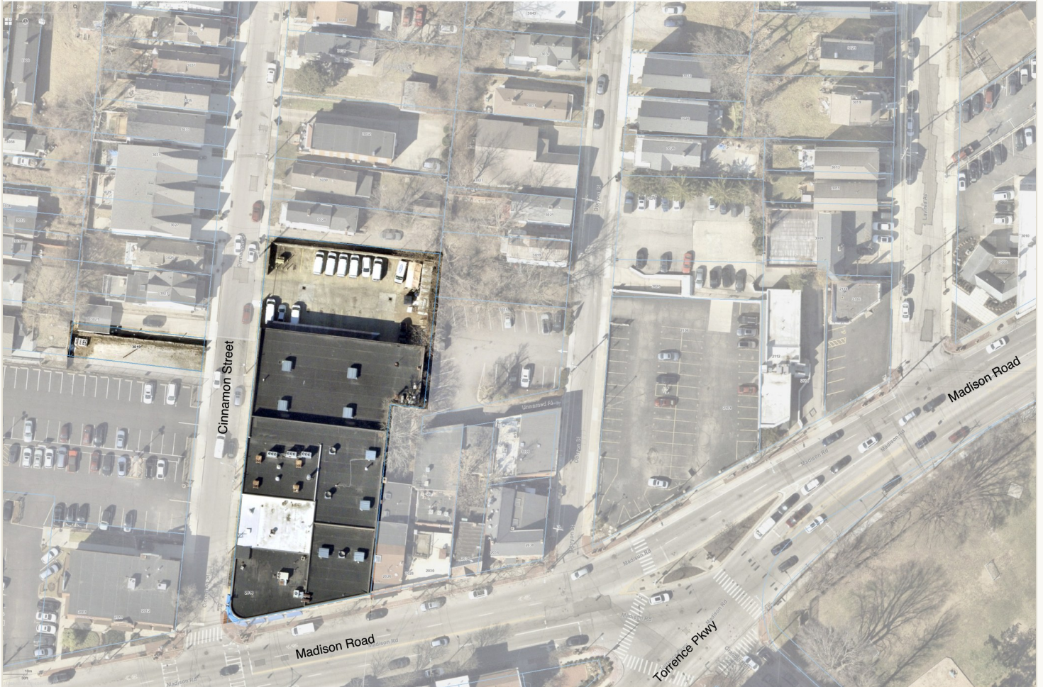
Madison Road corner at Cinnamon Street
