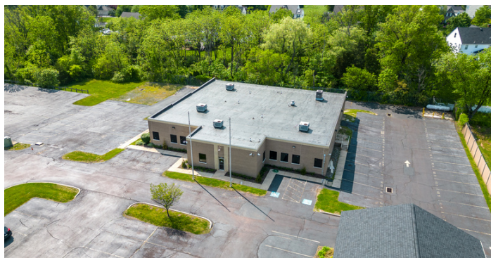
BUILDING B TOTAL SF: 9,200 RENT: $16/PSF (MODIFIED GROSS) NOTE: THIS RENT ASSUMES A FULLY AS-IS DELIVERY
