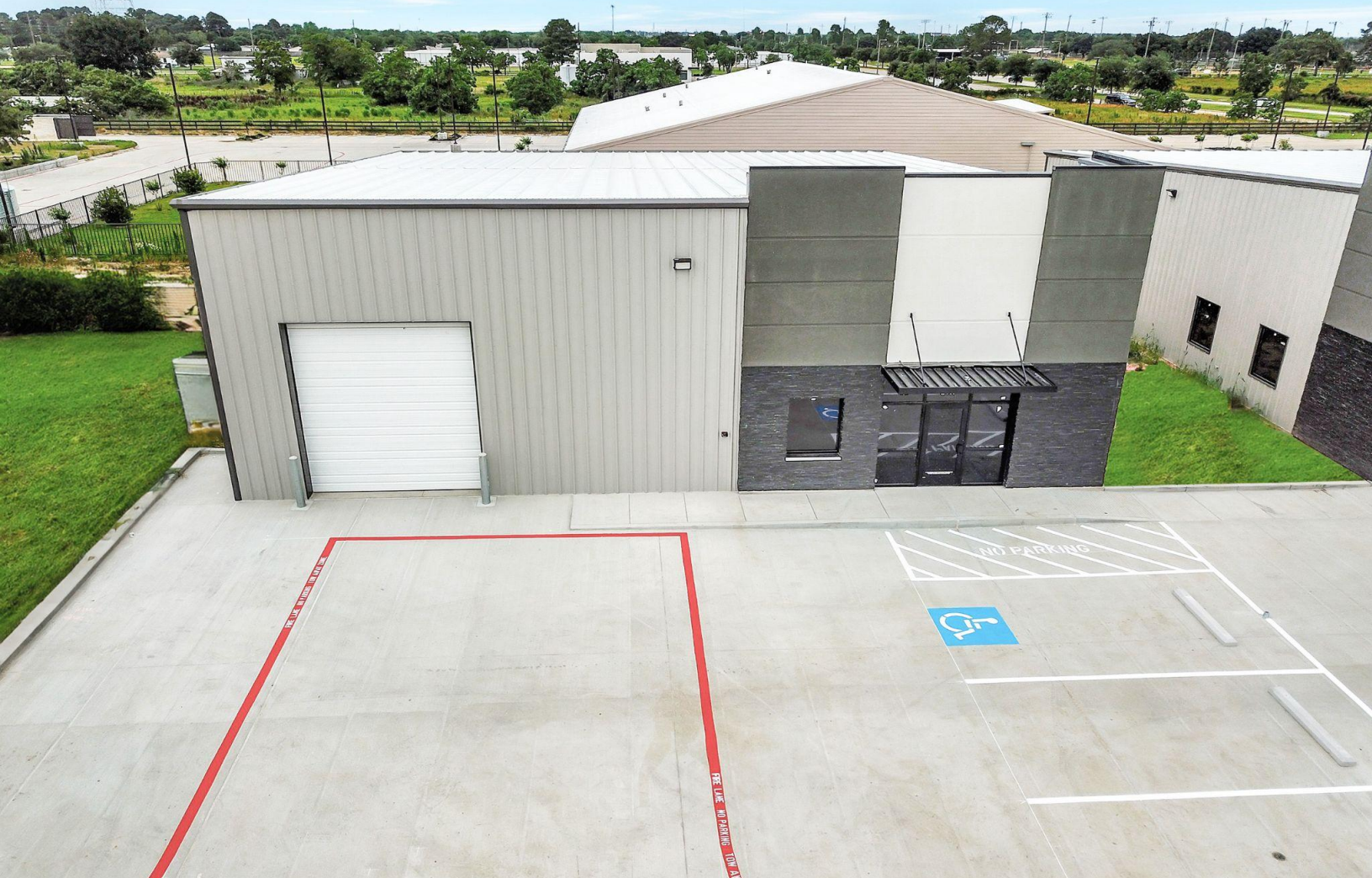
Exterior View of the Facility
