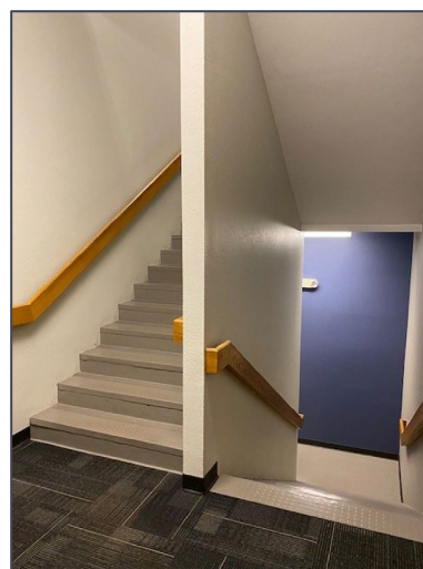
Stairway to Basement
