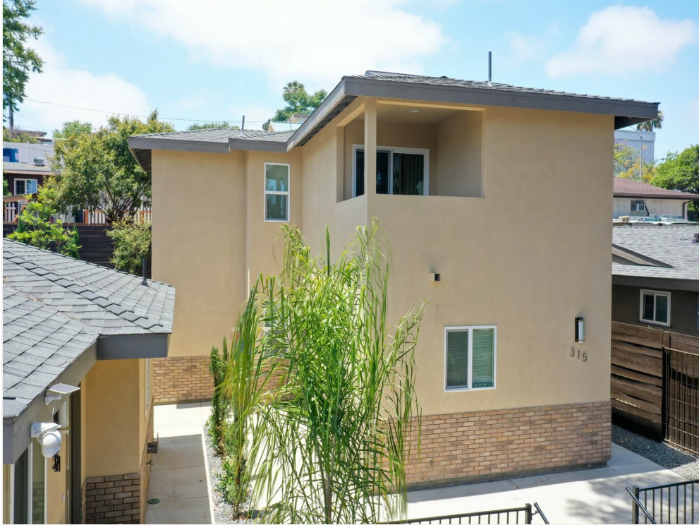
Exterior View of the Building
