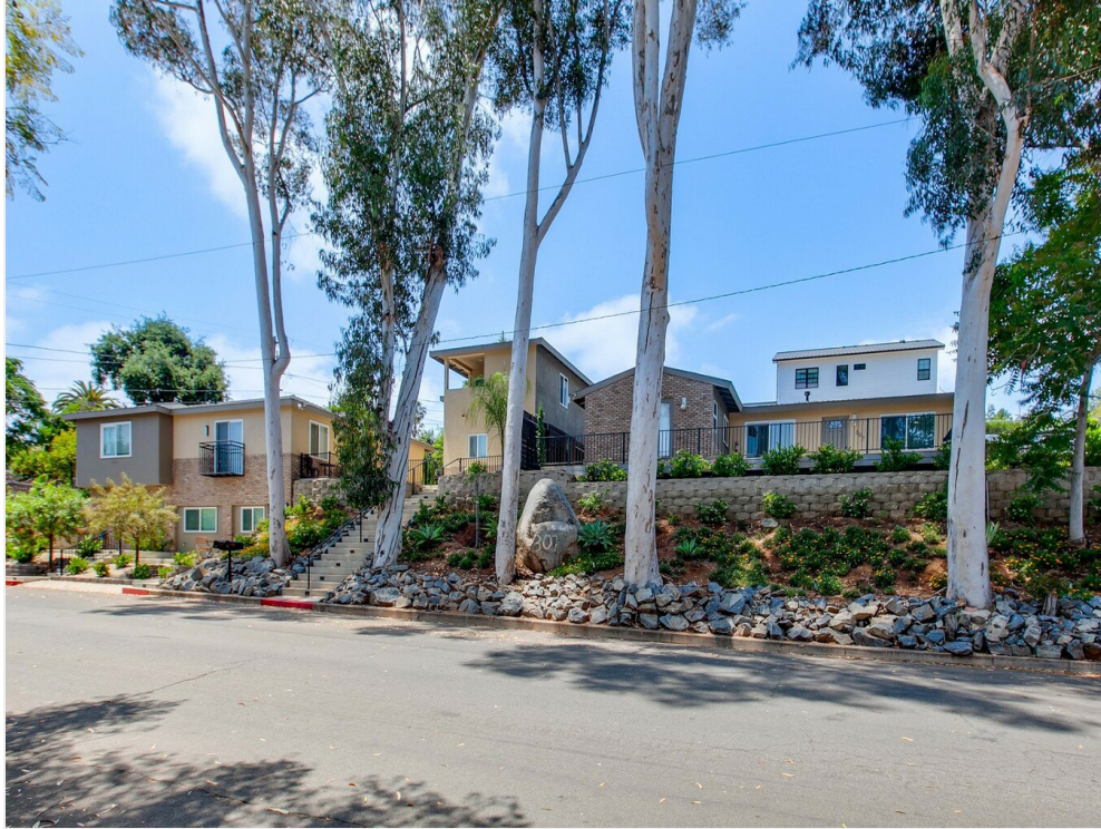
Exterior View of the Building
