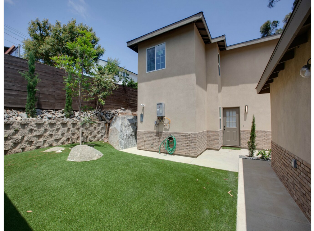
Exterior View of the Building
