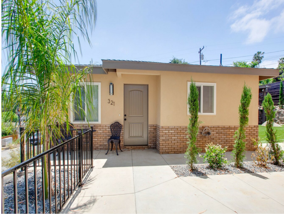
Exterior View of the Building
