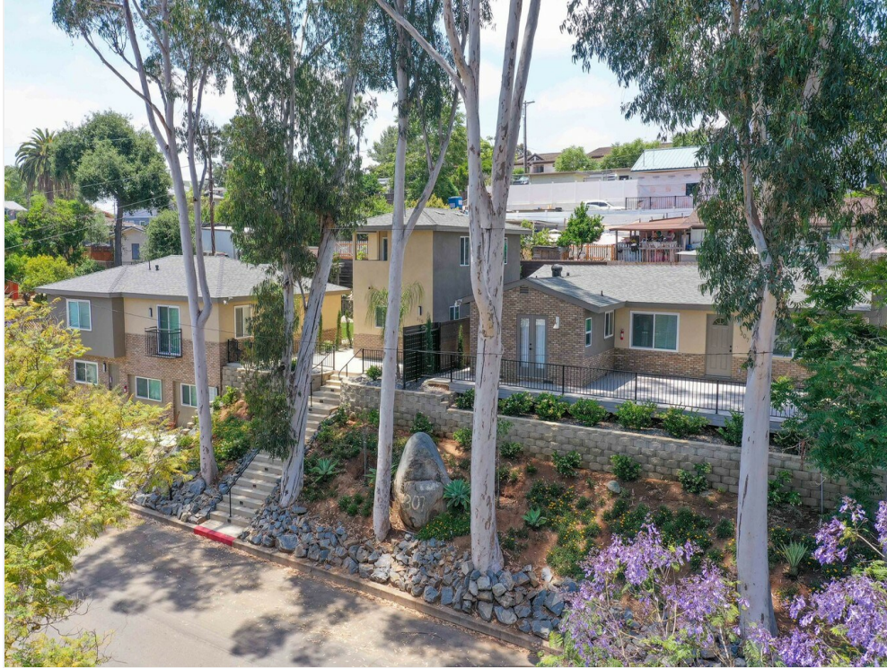
Exterior View of the Building
