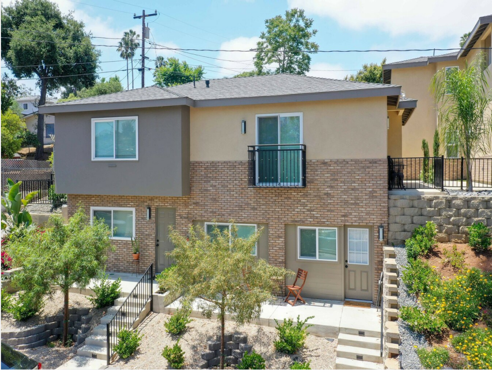
Exterior View of the Building
