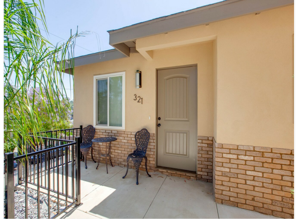
Exterior View of the Building
