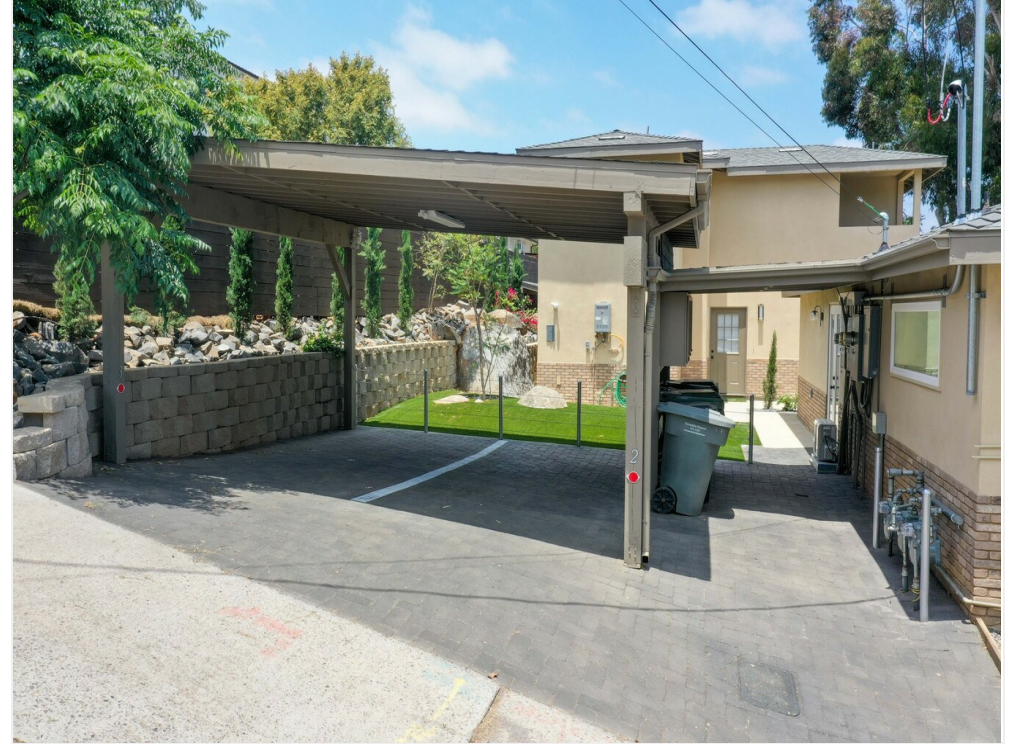
Exterior View of the Building
