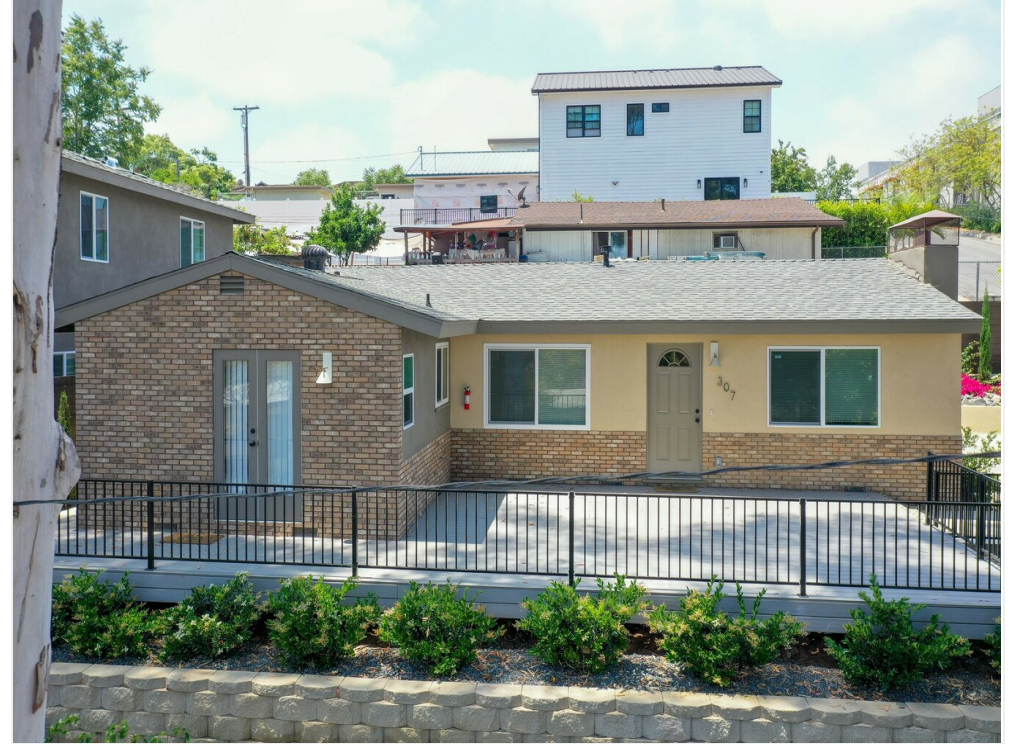
Exterior View of the Building
