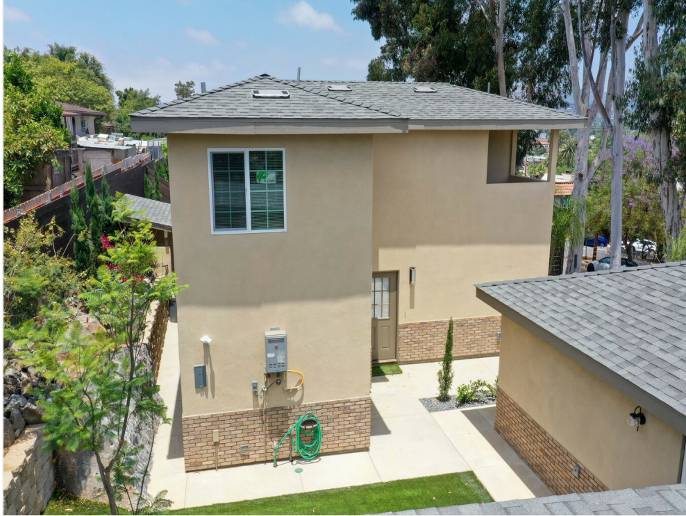
Exterior View of the Building
