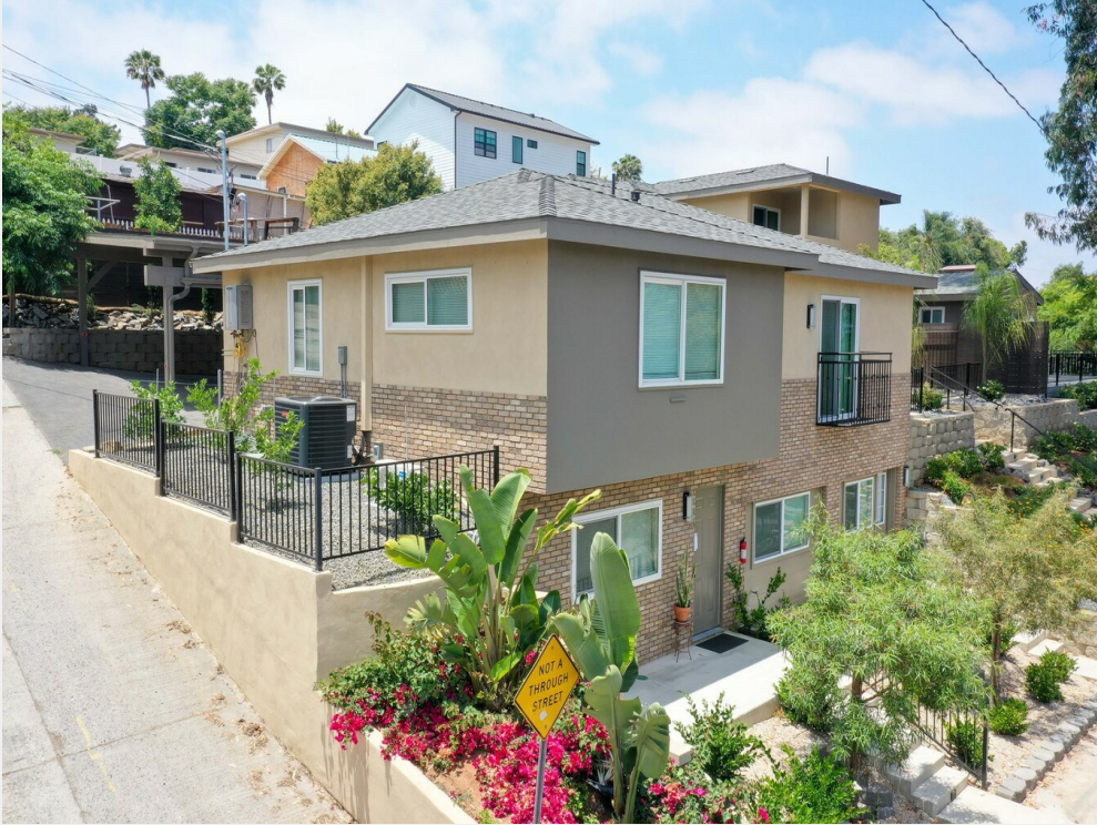
Exterior View of the Building
