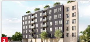
86 APARTMENTS 5547 N Elmer Ave
