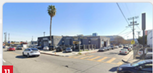
100 Apartments 11044 Burbank Blvd
