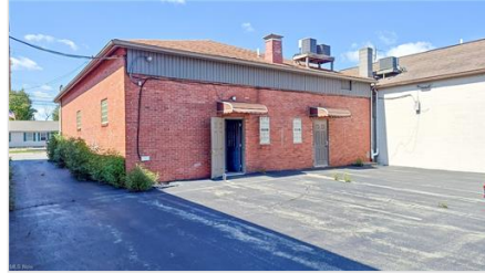
Back of Structure
