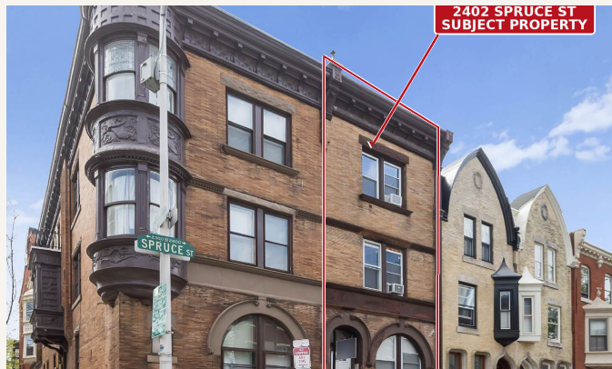
2402 SPRUCE STREET - SUBJECT PROPERTY
