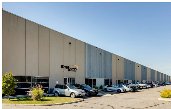
Airport Business Park - Building E
