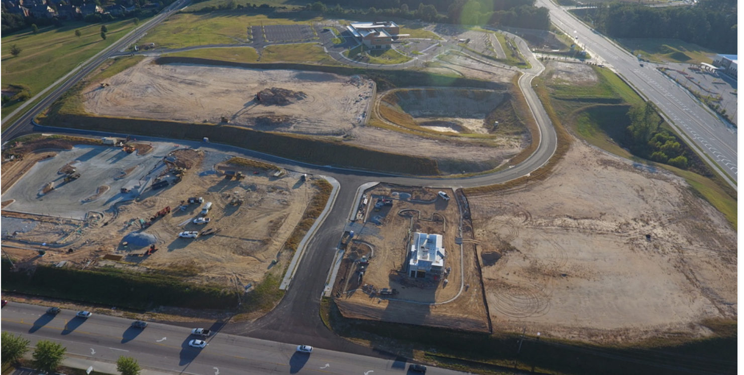
Graded Pads South Site
