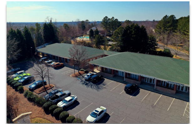
OFFICES AT VILLAGE PARK
