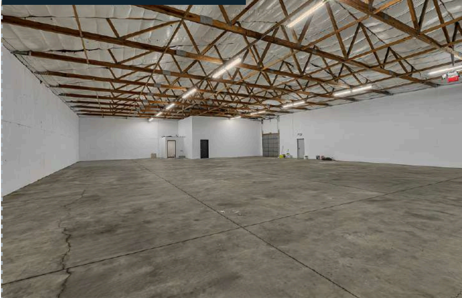
Unit 585: Working Area
