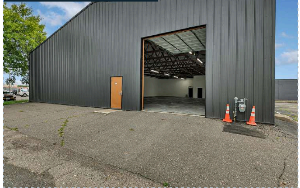
Unit 585: Drive in & Gas Meter
