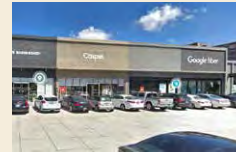
VARIOUS PAINT ACROSS FACADE
