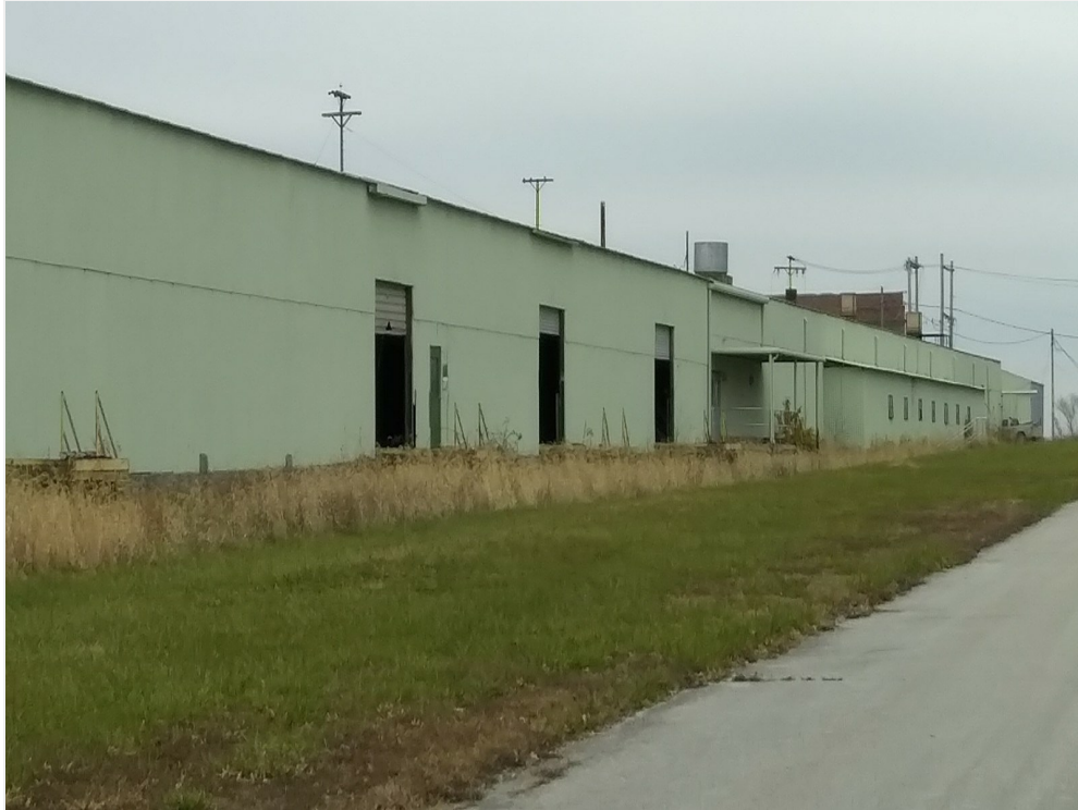
Rail Dock Doors
