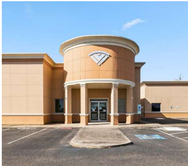
East Main Entrance
