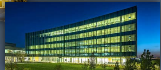
Anadarko Petroleum Building
