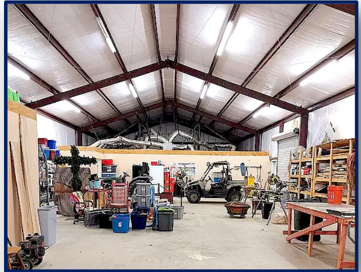
Warehouse/Shop 2 Storage Areas
