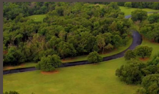
Private asphalt driveway through the property
