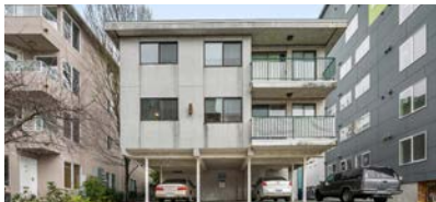
BALLARD COMMONS 5-UNIT 2232 NW 58th St
