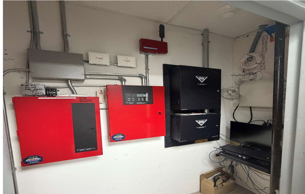
New fire alarm control panel
