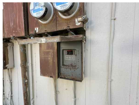
Exterior Main Shut Off Breaker
