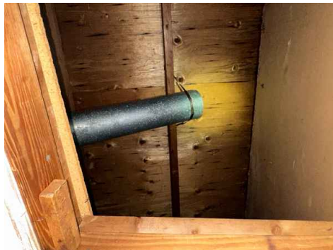
Appears to be a bathroom fan venting inside the attic
