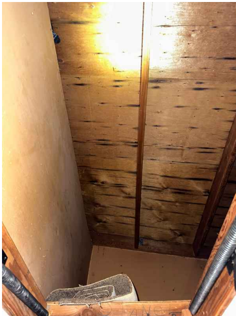
Appears to be a bathroom fan venting inside the attic
