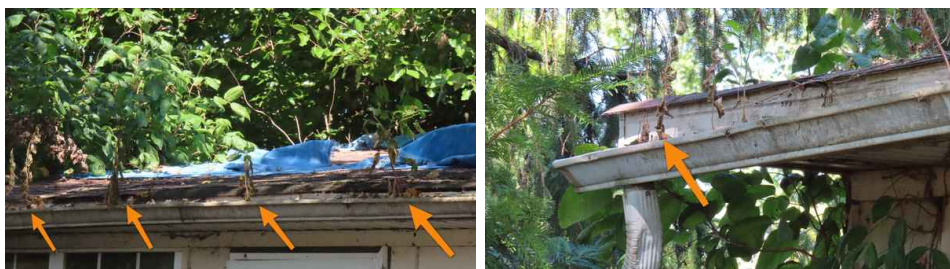
Weight of vegetation pulling gutter down
