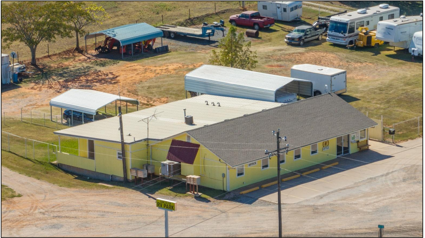
Photo 3: Aerial of The Office/Managers Residence
