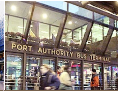
Port Authority Bus Terminal
