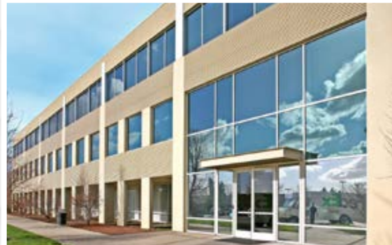
BUILDING E (EXPLORE) 10850 GOLD CENTER DRIVE
