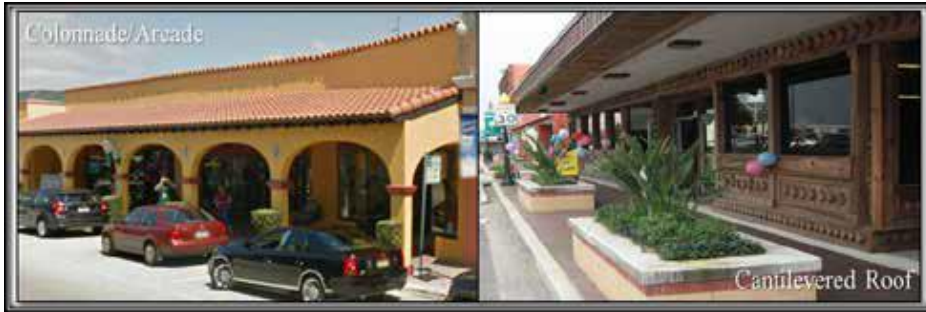
Figure 2.20 Colonnade, Arcade, Cantilevered Roof
