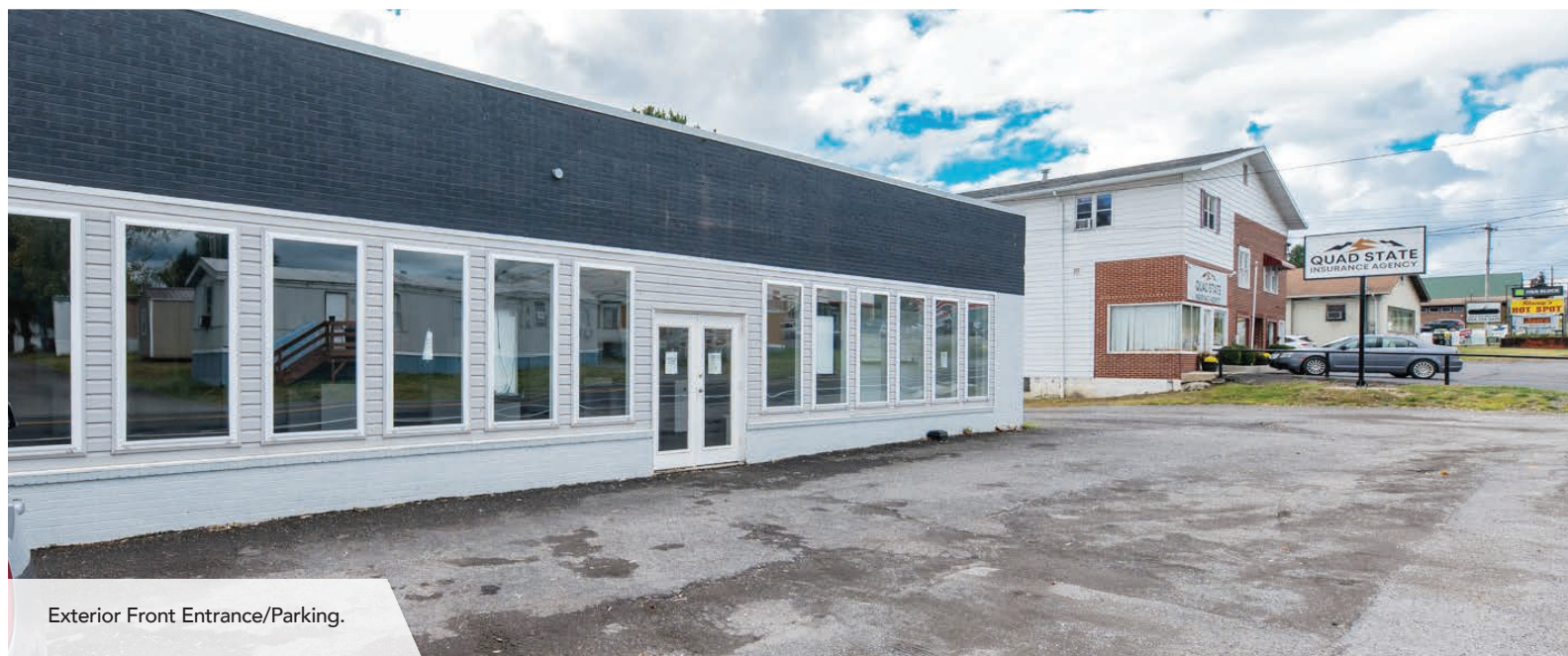
Exterior Side/Entrance to Warehouse Space.
