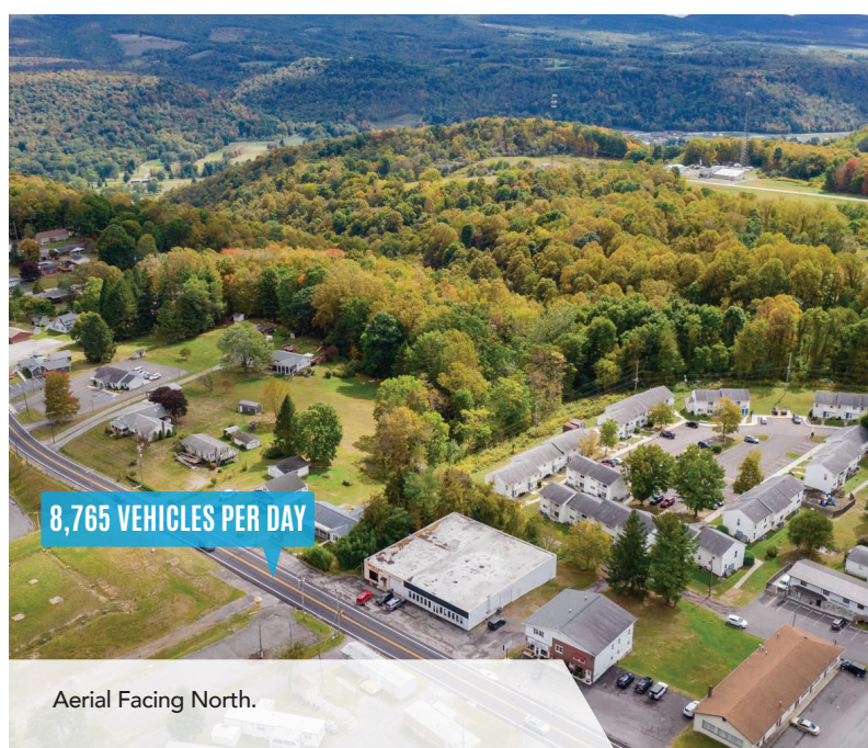
Aerial Facing North.
