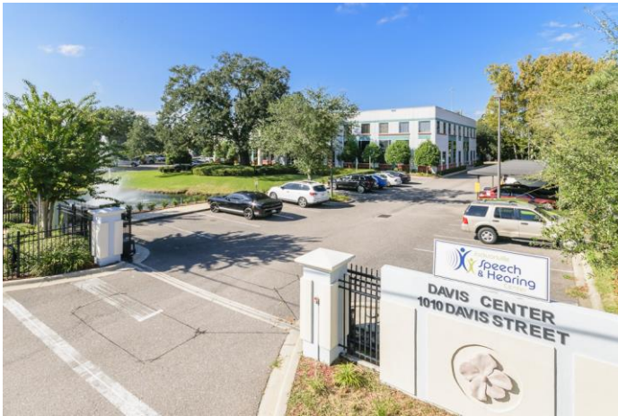
Secured Entrance (Right)
