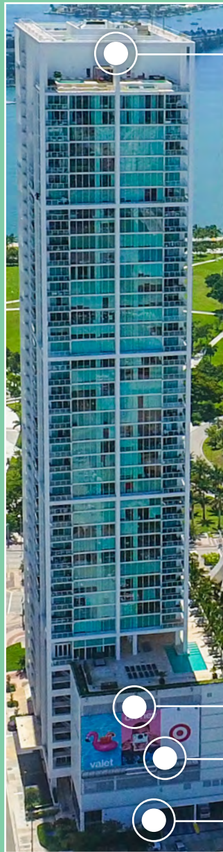
VIEW FACING WEST
