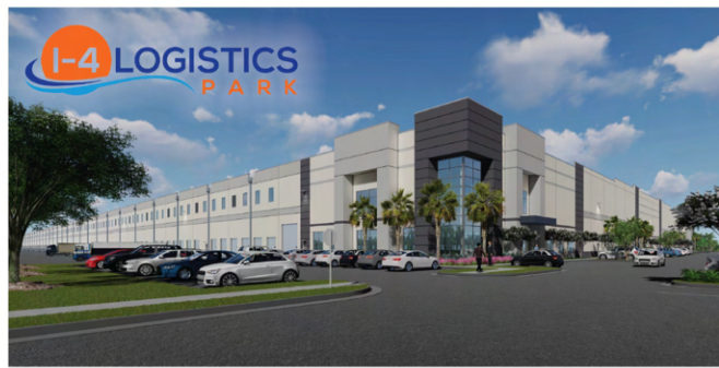
I-4 Logistics Park - .33 Mi Under Construction
