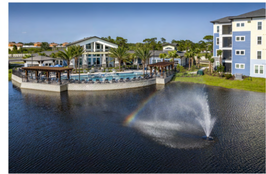
Integra Myst - .92 Mi 300 Apt. Units Under Construction
