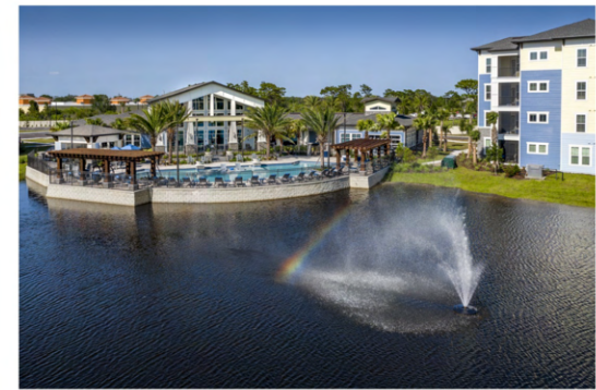
Integra Myst - .79 Mi 300 Apt. Units Under Construction
