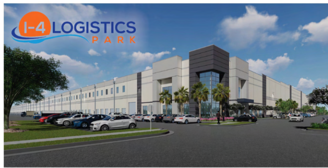
I-4 Logistics Park - .24 Mi Under Construction
