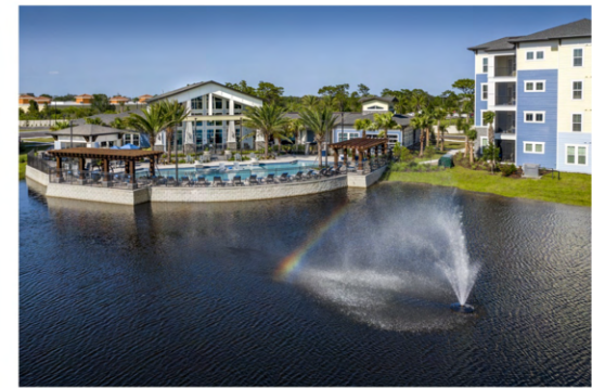
Integra Myst - .56 Mi 300 Apt. Units Under Construction
