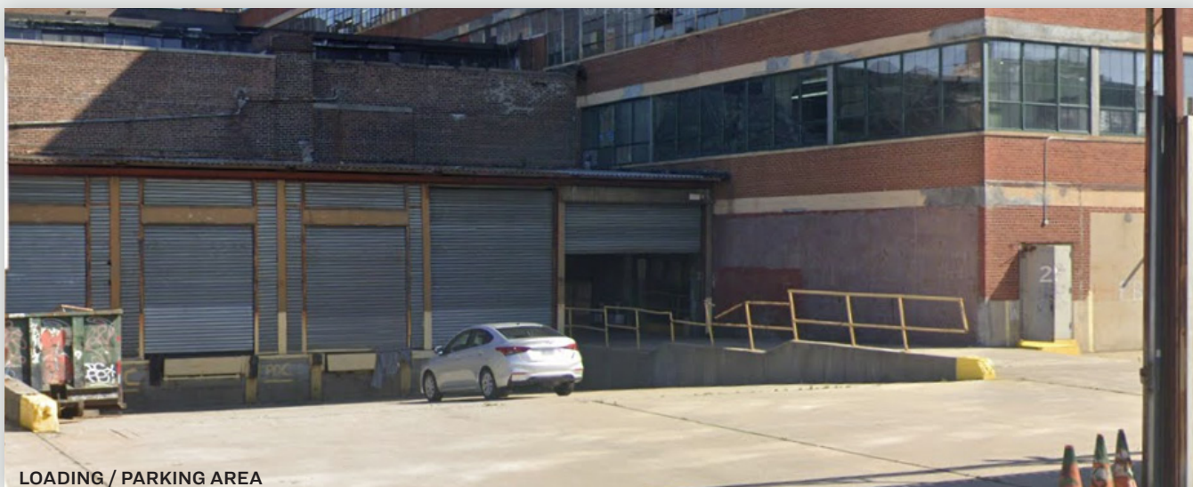
LOADING / PARKING AREA
