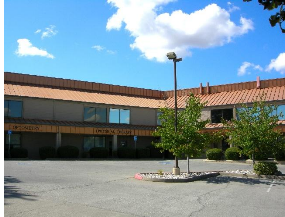
Front of building
