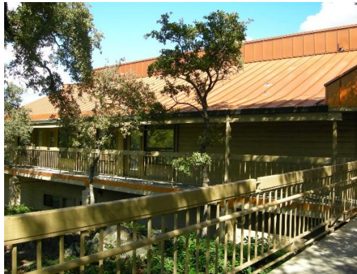
Ground level access to unit
