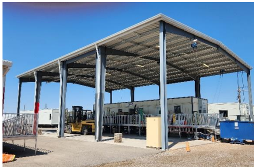
Covered workspace (canopy to remain; modular building not included)
