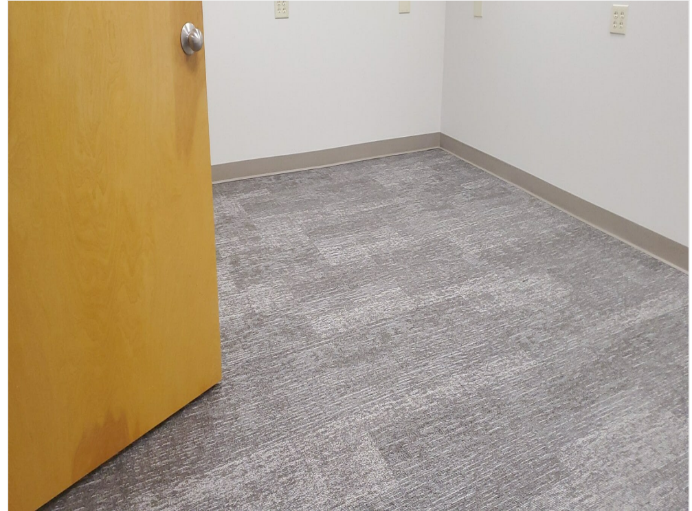
Renovated for new tenant
