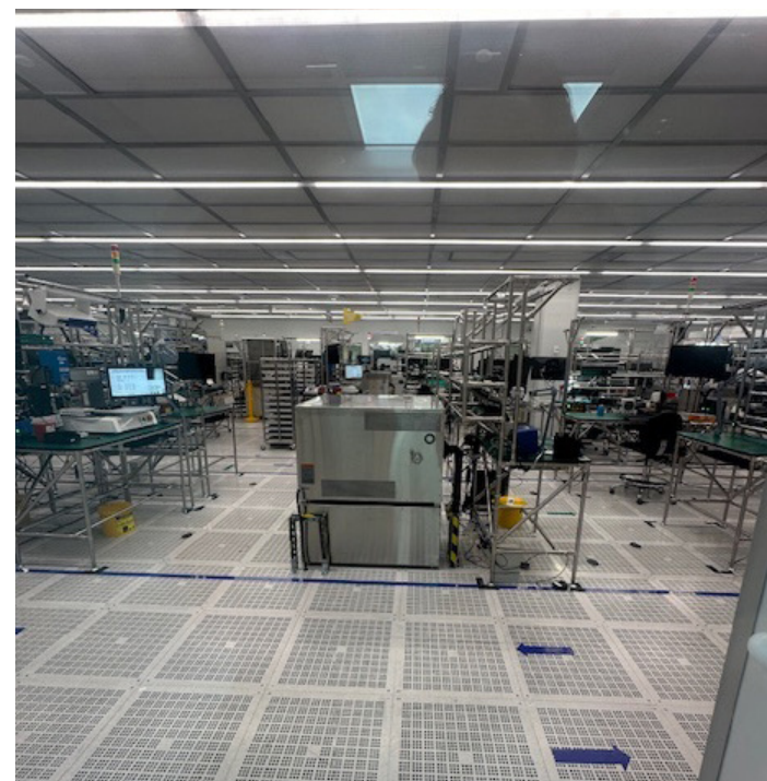
ISO 5 CLASS 100 CLEAN ROOM WITH RAISED FLOORS
